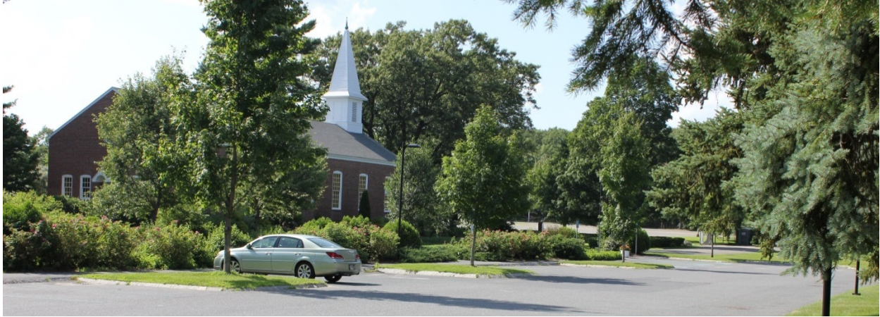
The 90 space parking area at Cushing Chapel was constructed in 2003, the first parking facility designed to support the new passive park development.
